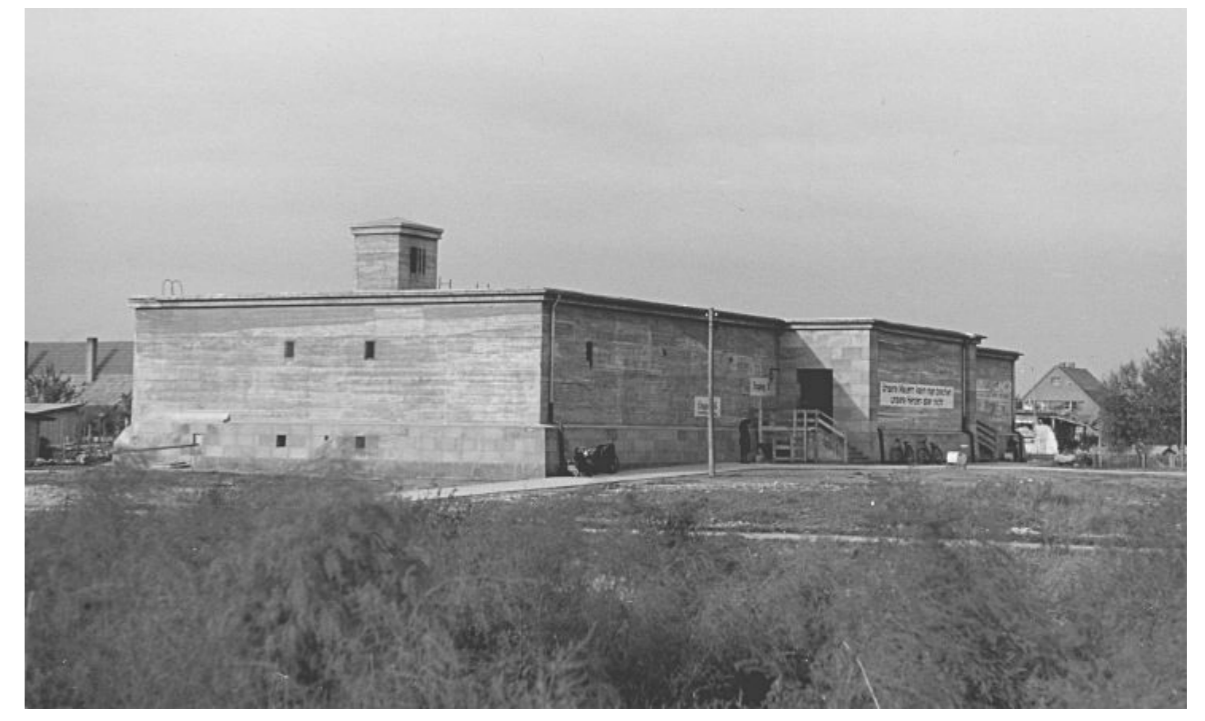
Photo Speckwegbunker after completion, MARCHIVUM „KF01909“
